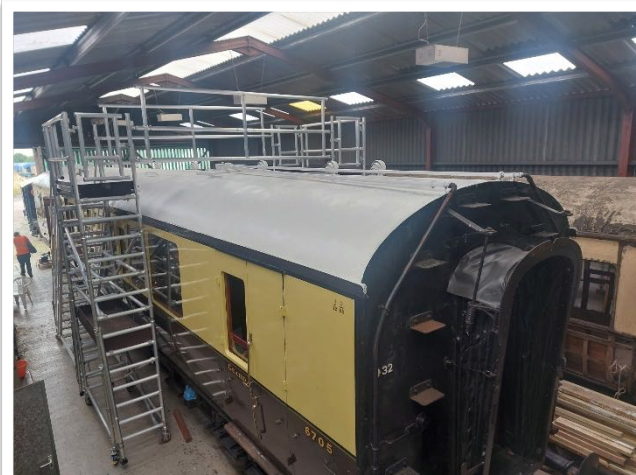
Painting of 6705's roof has been completed
