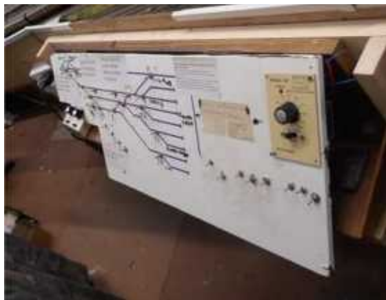
Above is a picture of the old Shunting Yard panel that has been in place for many years.
