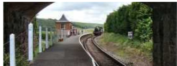
The trackwork at Doniford.
