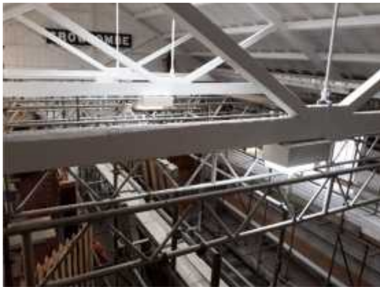
The scaffolding inside the museum is finally being removed.
