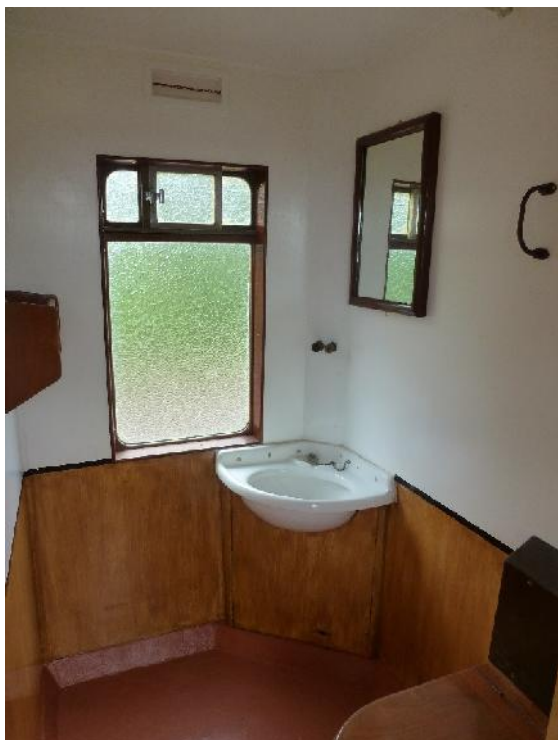
(BCK 6705 - the toilet has only just been completed.)
