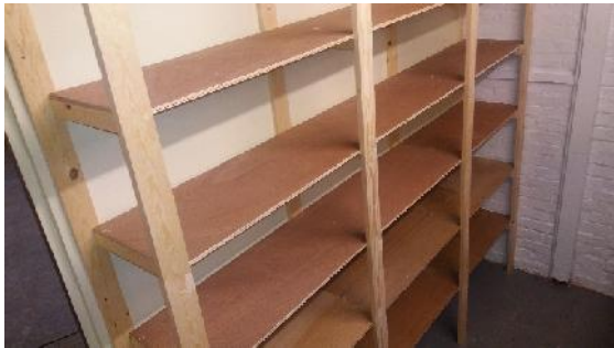
New shelving being erected in the Store extension
